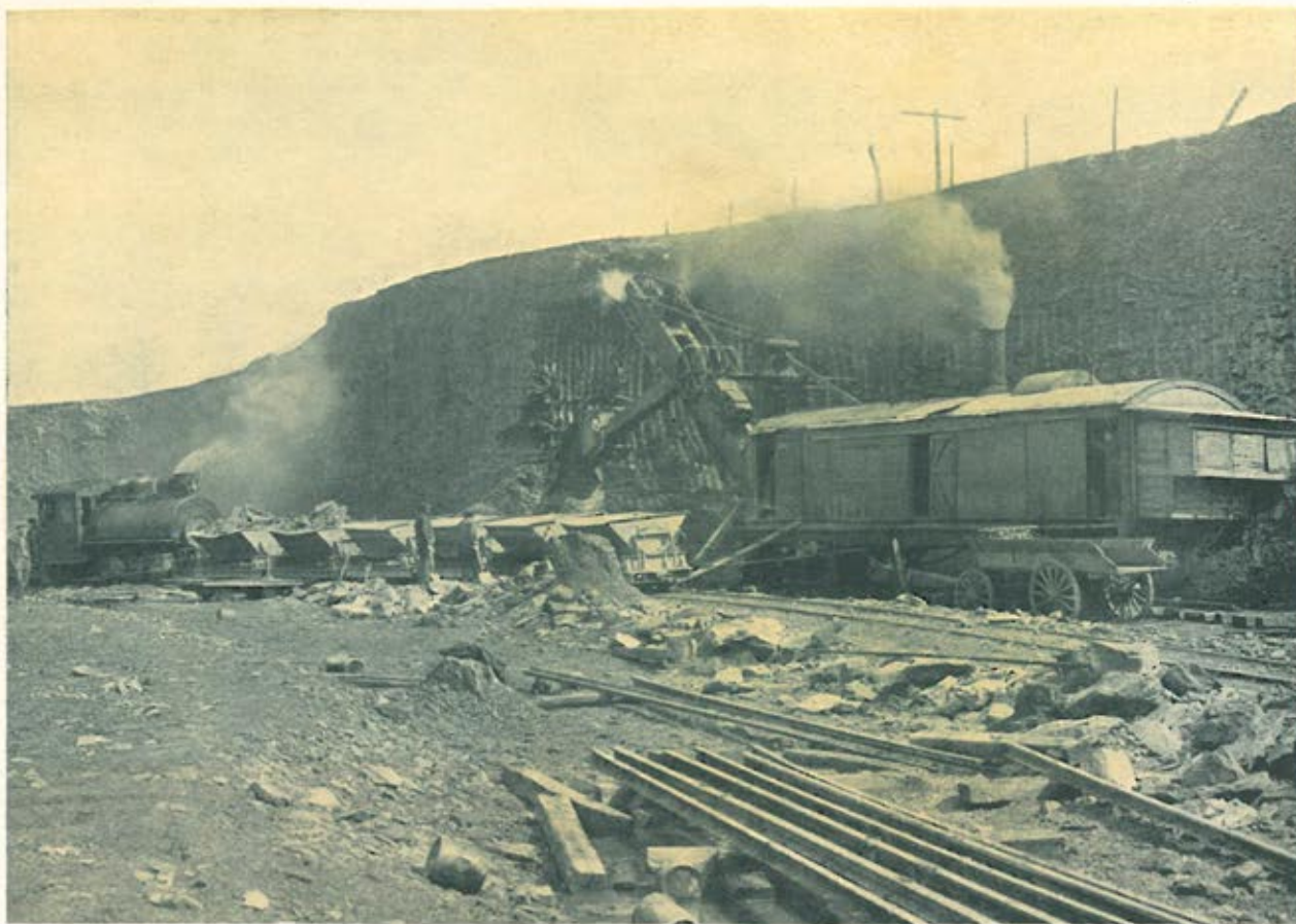
Steam Shovel at work on Shale bank.
