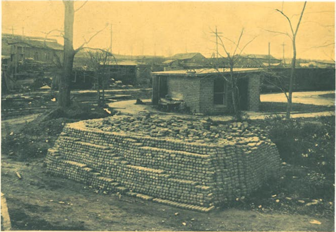
Brick which have passed through the Rattler Test. Note their uniformity. The Rattler Shed is behind the pile.
